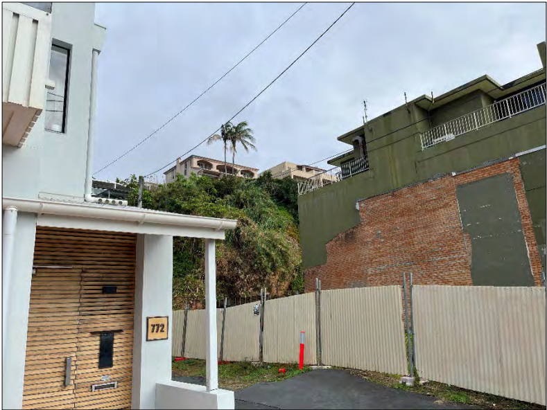
Figure 5 – View of subject site from road frontage.
