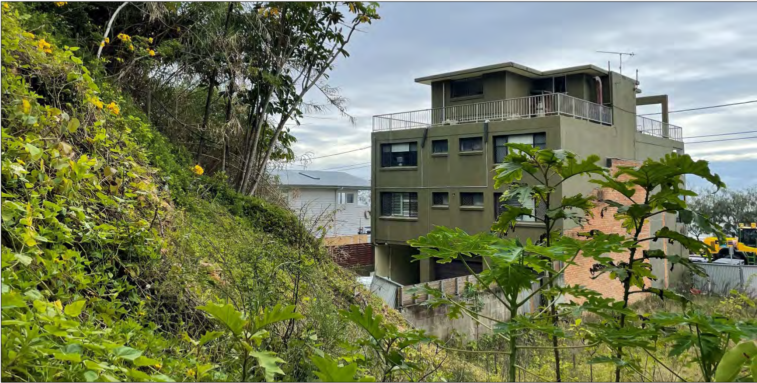
Figure 2 – View to the east from the rear of the property.
