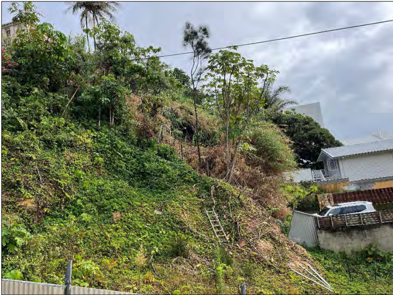
Figure 4 – View of the slope at the rear of the property.
