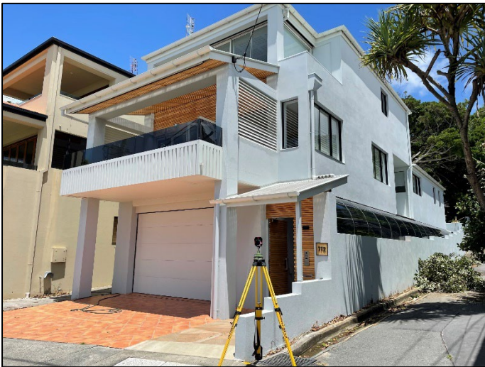
3 storey dwelling at 772 Pacific Parad
