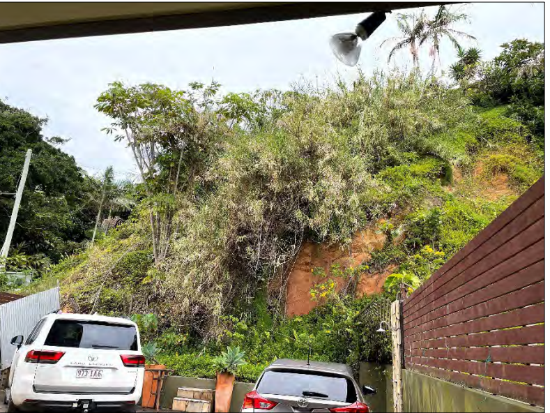
Figure 6 – View of the slope at the rear of the property.
